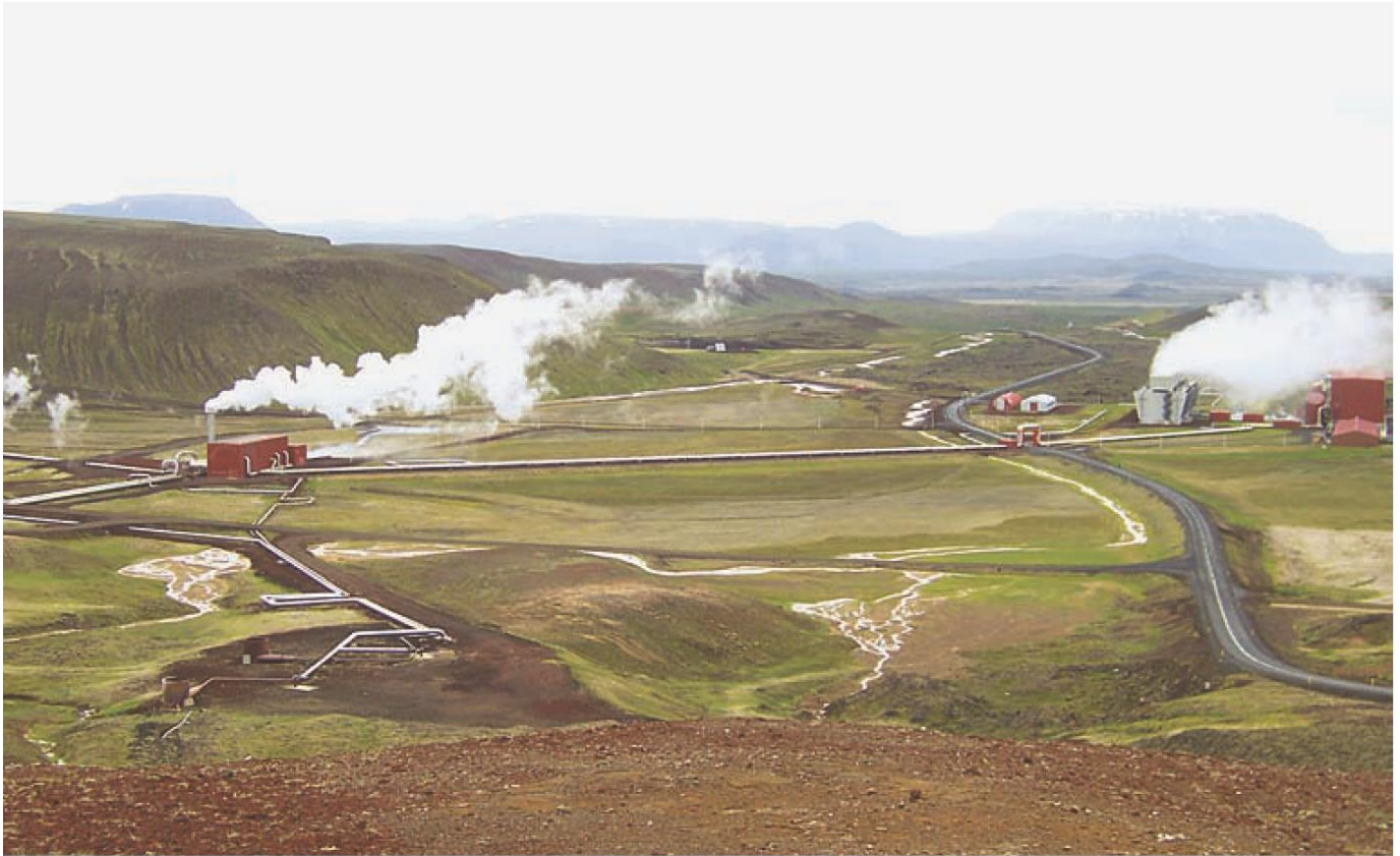
Krafla Geothermal Station in northeast Iceland. Despite having the richest geothermal resources in the world, in Iceland most electricity is generated with hydroelectric power. (Mike Schiraldi)
