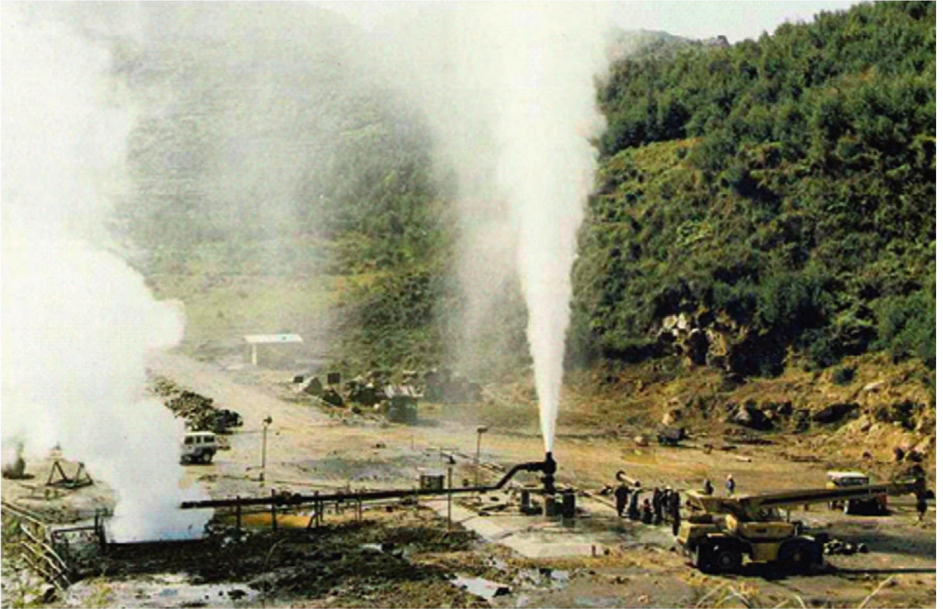
Fig. 3.2 Initial blowing of an Indonesian well at the Dieng geothermal field [1] [WWW].
