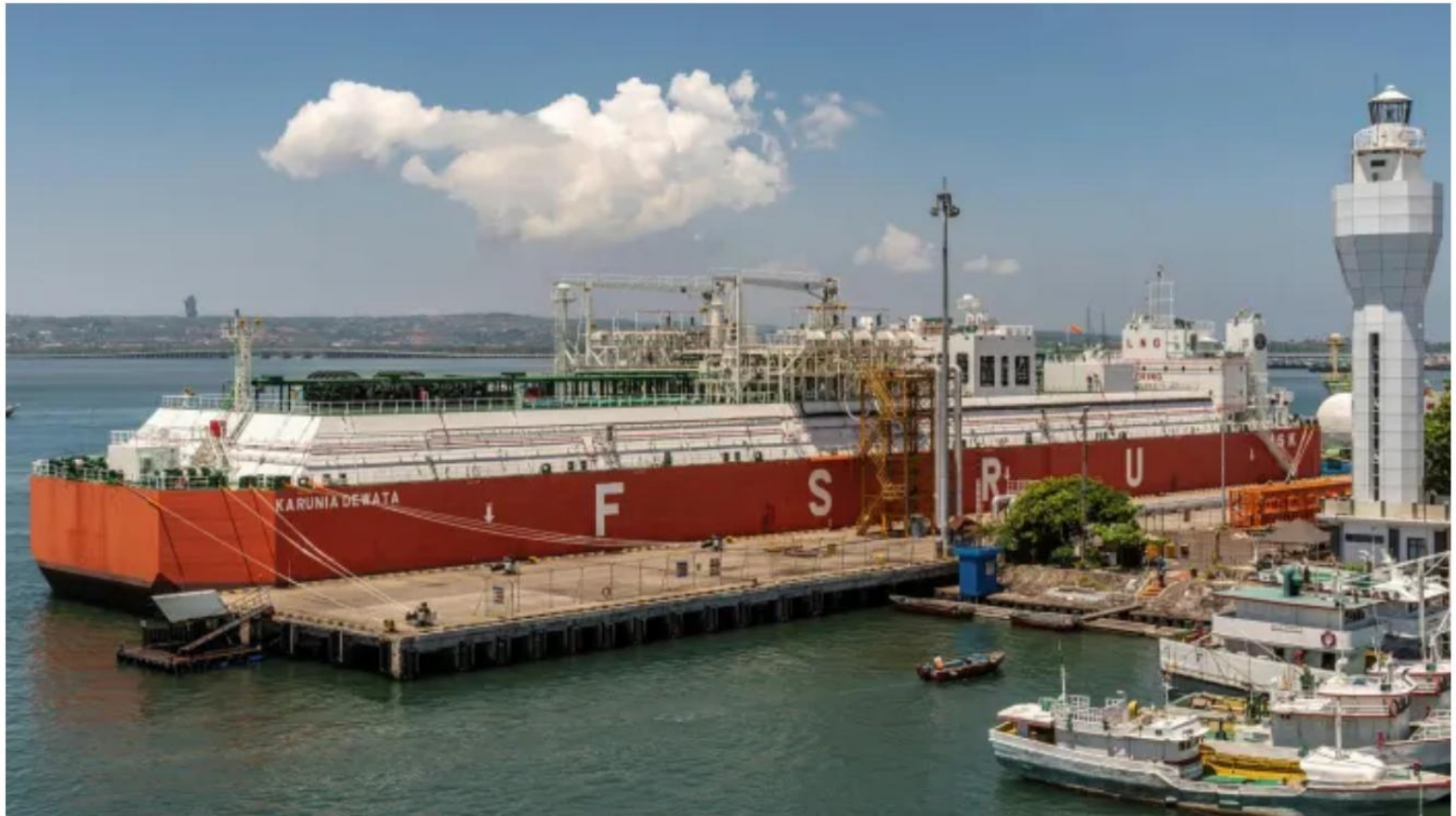
A floating storage and regasification unit. The ships offer the fastest way for Europe to boost LNG imports © Claudine Klodien/Alamy
