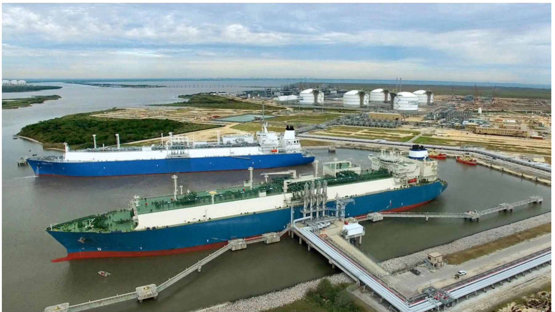
Ships at Cheniere Energy's Sabine Pass terminal being loaded with liquefied natural gas. Cheniere
