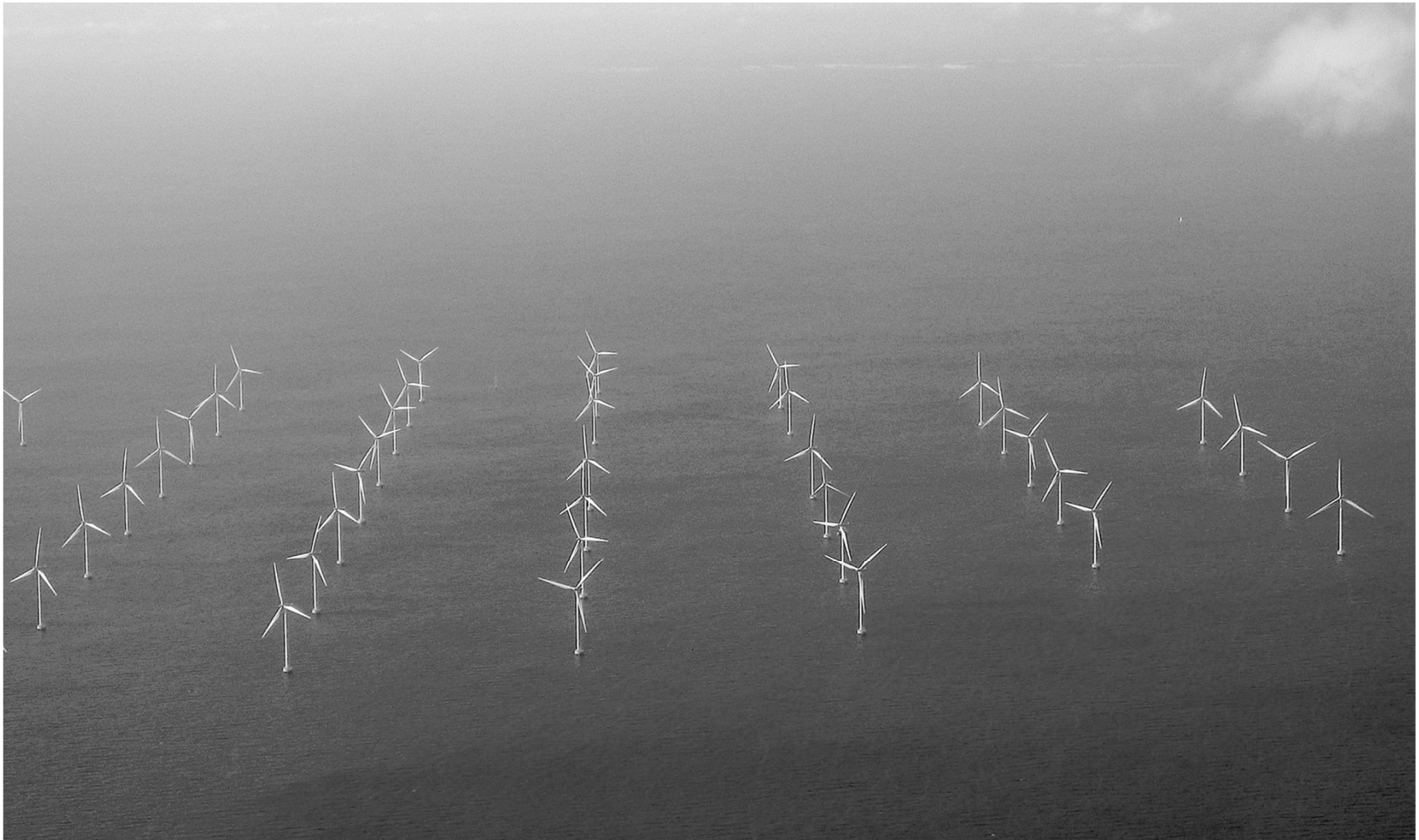
An Off-Shore Wind Power Plant in the Netherlands.
