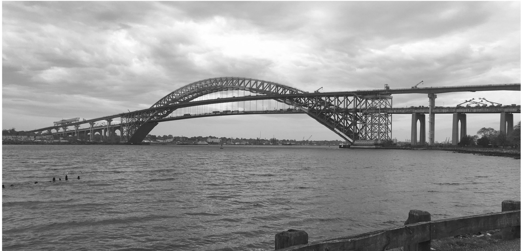
The Bayonne Bridge's Deck was raised from 155 feet (47m) to 215 feet (66m). Port of New York Source: Arnold Reinhold
