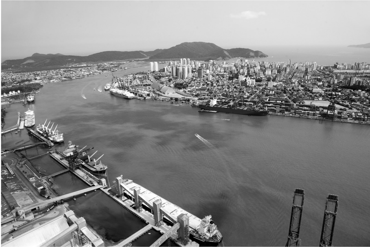
The Port of Santos in Brazil, limited by the growth of the city, and the width of the river Source: Luis Inácio P Prado
