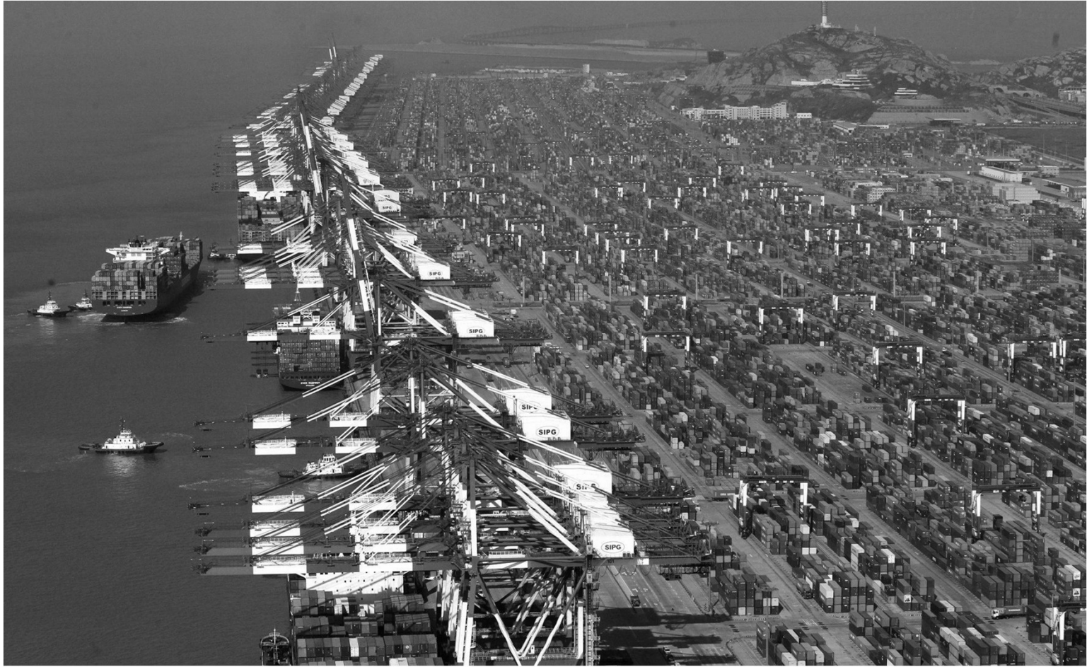
The Port of Yangshan was created because the Port of Shanghai did not have enough water draft Source: Port of Shanghai Authority
