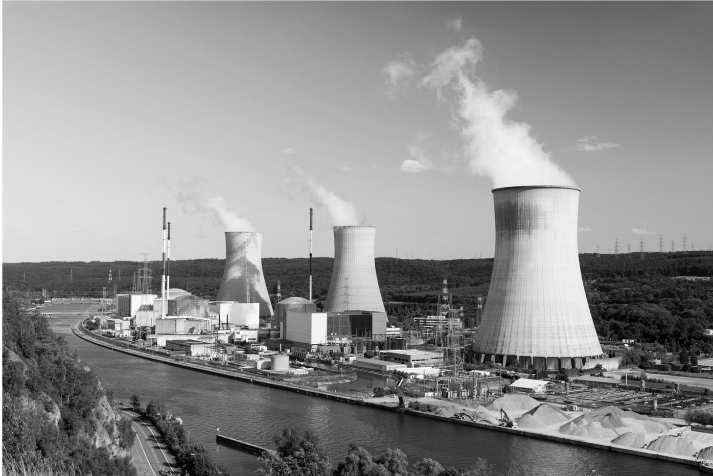
Nuclear Power Plant in Tihange, Belgium.
