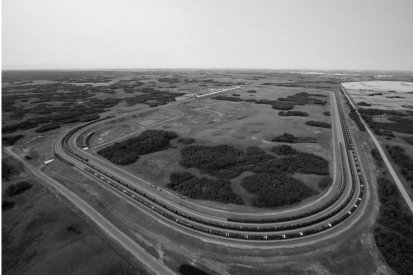
The Hardisty Oil Terminal in Alberta, Canada, where oil is loaded onto trains that take the oil to the Cushing Terminal in Oklahoma, in the United States, where it is transferred to the pipeline network. Source: USD Partners LP
