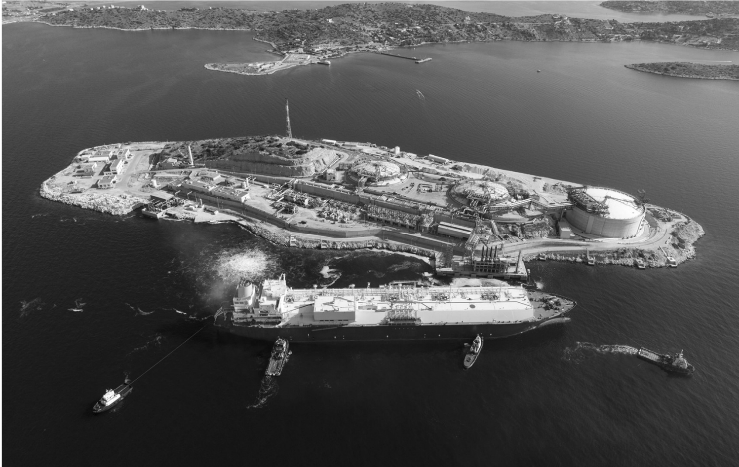
The LNG import terminal in the Port of Revithoussa in Greece. Source: DESFA
