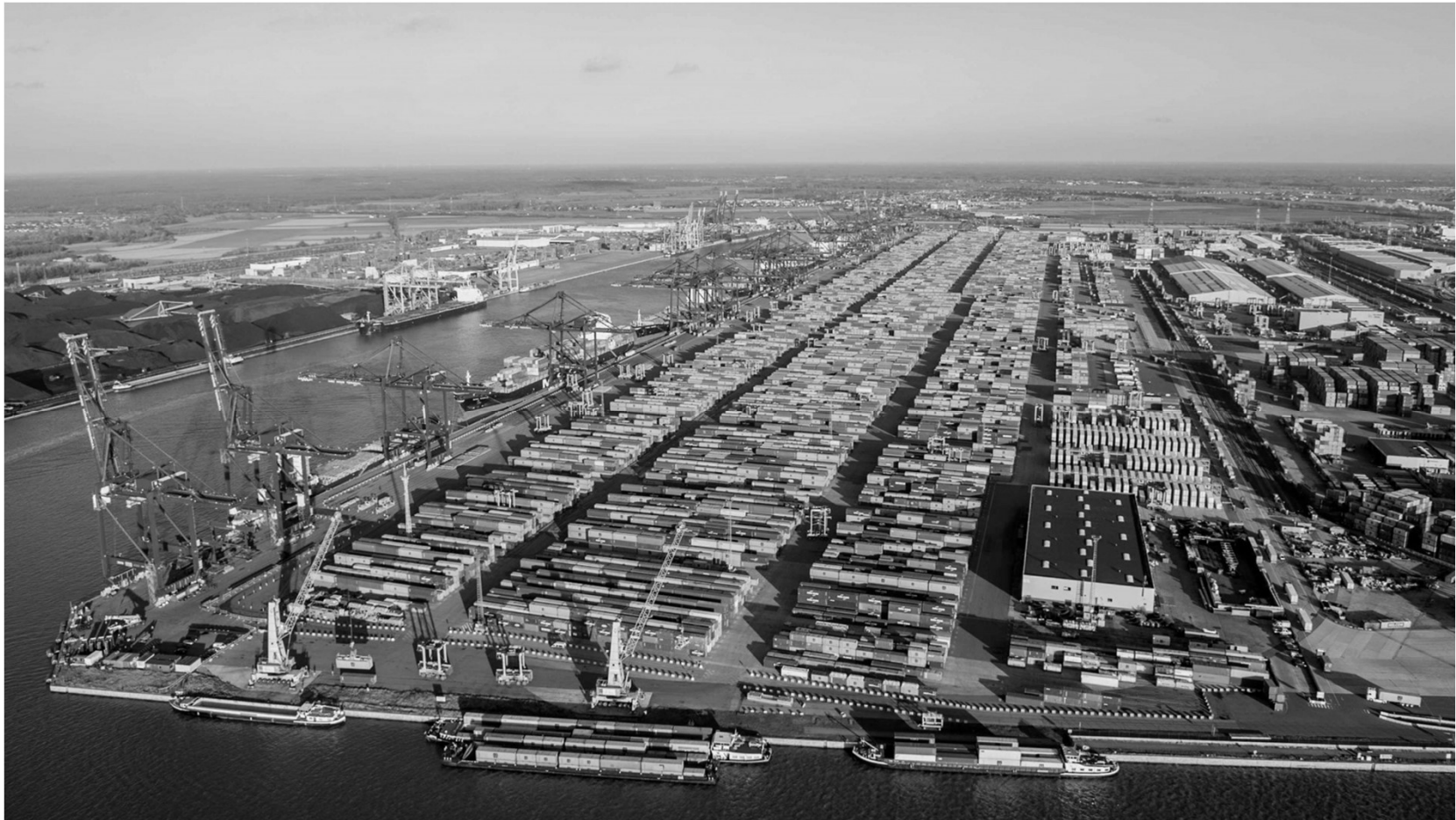
The container yard area in the Port of Antwerp . Source: PSA Antwerp
