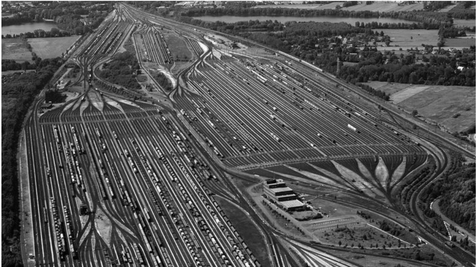
The Maschen Hamburg rail yard in Germany assembles trains with railcars from different origins. Source: pa/dpa
