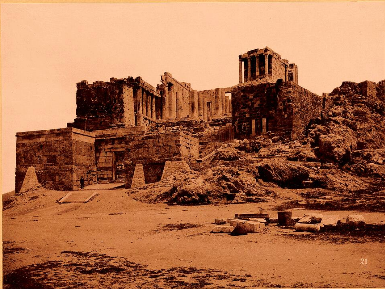
Beulé Gate 5 1/2 ft wide excavated 1853 by French savant Beulé. Date erection uncertain but of late period. Bastions Turkish.
