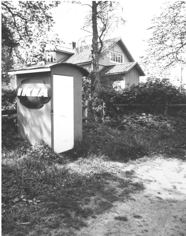
This tiny shed in Sweden is where Ingvar stored his first lot of IKEA packages.
