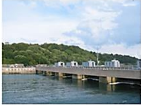
Barrage of the tidal power plant on the estuary of the Rance River in Bretagne, France Source: Stock photography (copyrighted)
