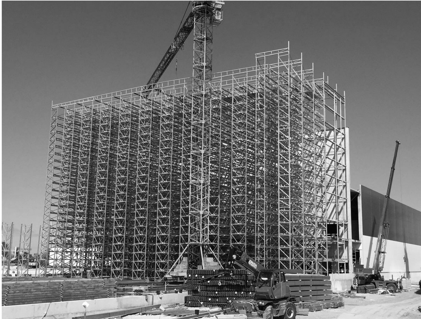
A very high-bay warehouse under construction in Germany Source: Voestalpine
